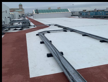
Finished Top Coat with Walkway
