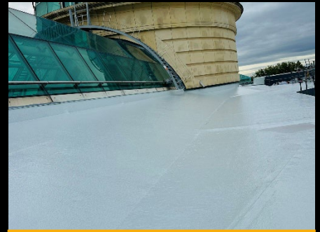
Finished Top Coat
