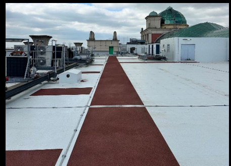
Finished Top Coat with Walkway
