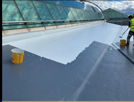
Top Coat Being Applied
