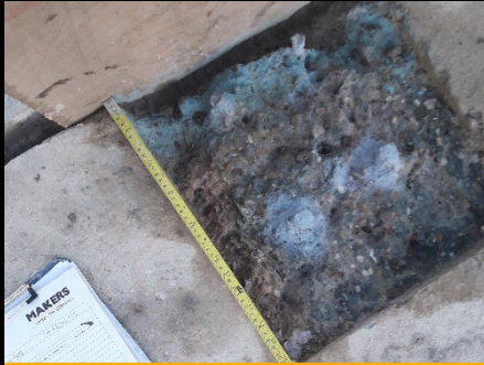
Concrete repair broken out
