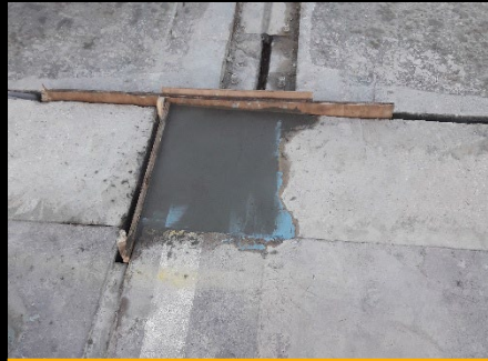
Concrete repair reinstated
