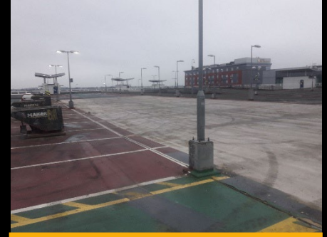
Area ready for captive blast
