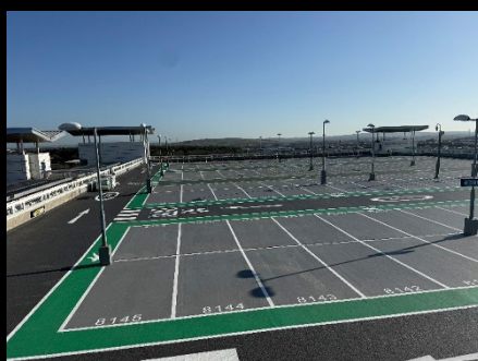
Works complete to phase 1 & 2
