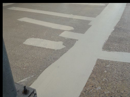
Reinforcement banding complete
