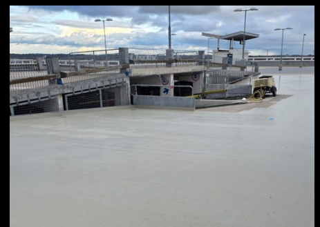
Area fully reinforced
