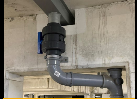
New shut off valve installed
