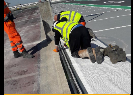
Installing the new expansion joint
