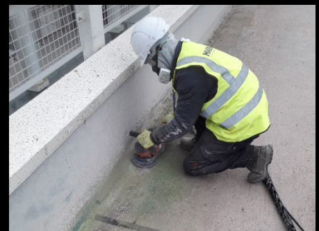
Edge preparation to
