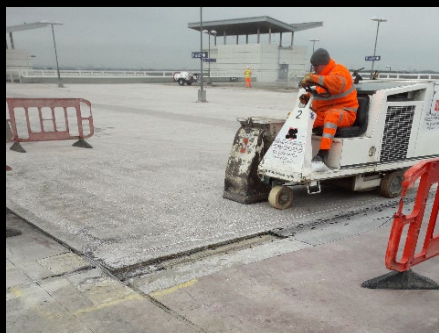
Captive blast being carried out
