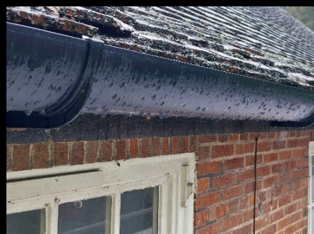
Preparation - New Guttering
