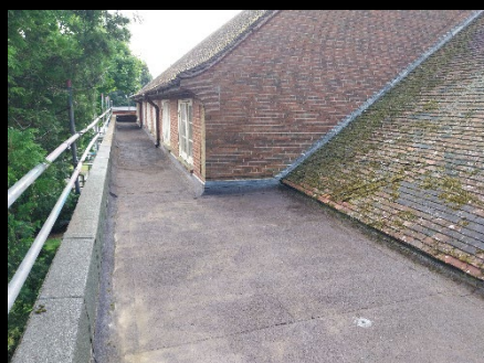
Preparation – Ready to strip up
