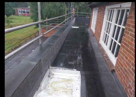
Preparation – New Insulation
