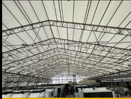
Central Roof – Temporary Roof
