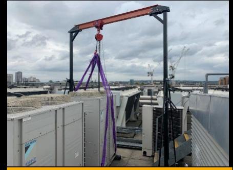
Central Roof – Plant Lifting
