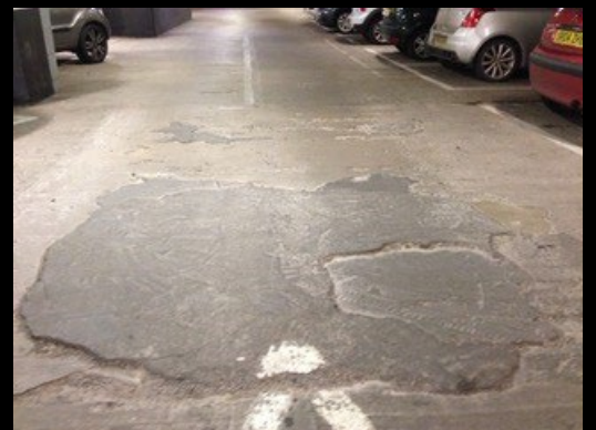
Multiple Failed Repairs
