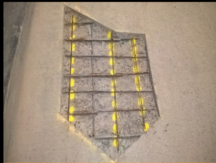
Replacement Reinforcement
