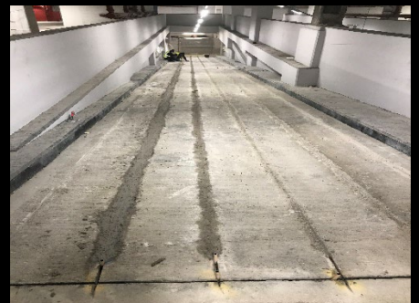
Conductive Mortar Anode
