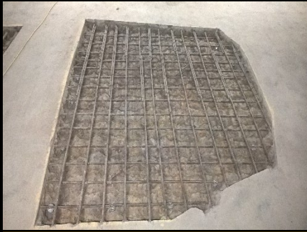
Excavated Repair
