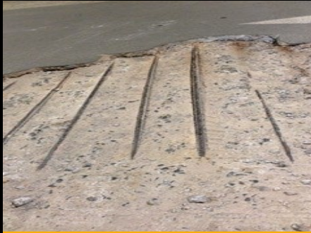
Exposed Surface Steel
