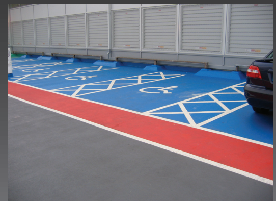
Triflex DFS external to asphalt
