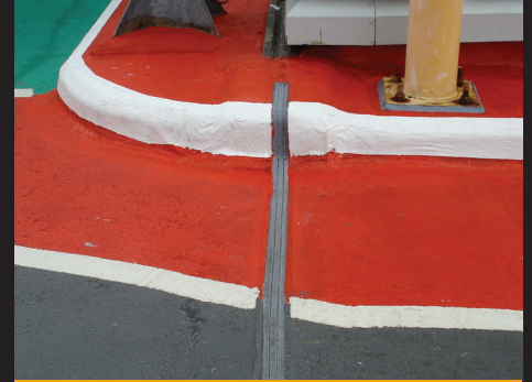
Emseal DSM installed
