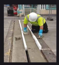
The asphalt was saw-cut 240mm either side of the failing pre-formed movement joints and removed to expose the concrete deck. The asphalt was also then cut back a further 100mm x 5mm deep. The main joint arrisses were re-formed with a rapid setting cementitious mortar & resin bonding agent 200mm wide x 40mm deep. The main movement joints were re-formed to 50mm wide in readiness for the new Emseal DSM joint.
