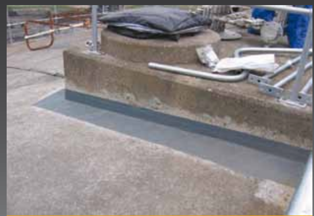
External joint sealing
