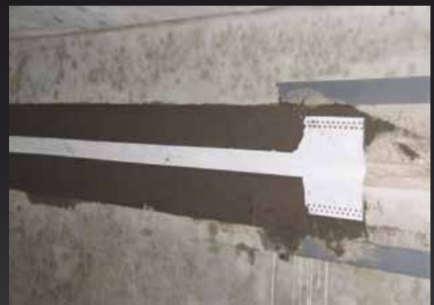
Internal flexible joint banding
