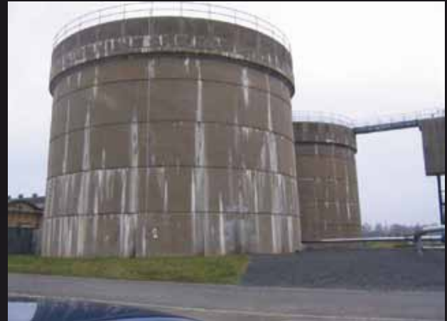
Typical concrete digester tank
